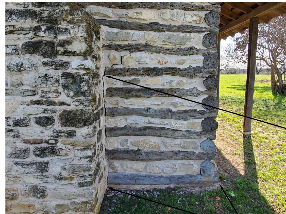
F SOUTH CABIN SW CORNER
