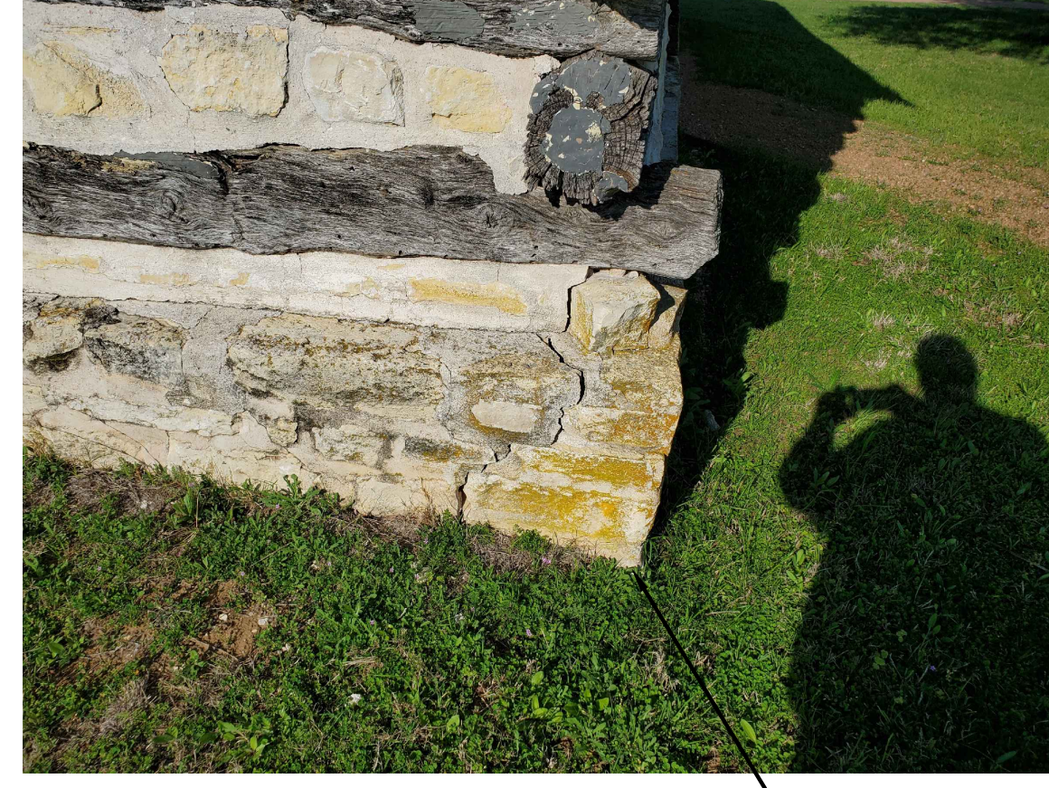
C NORTH CABIN NE CORNER
