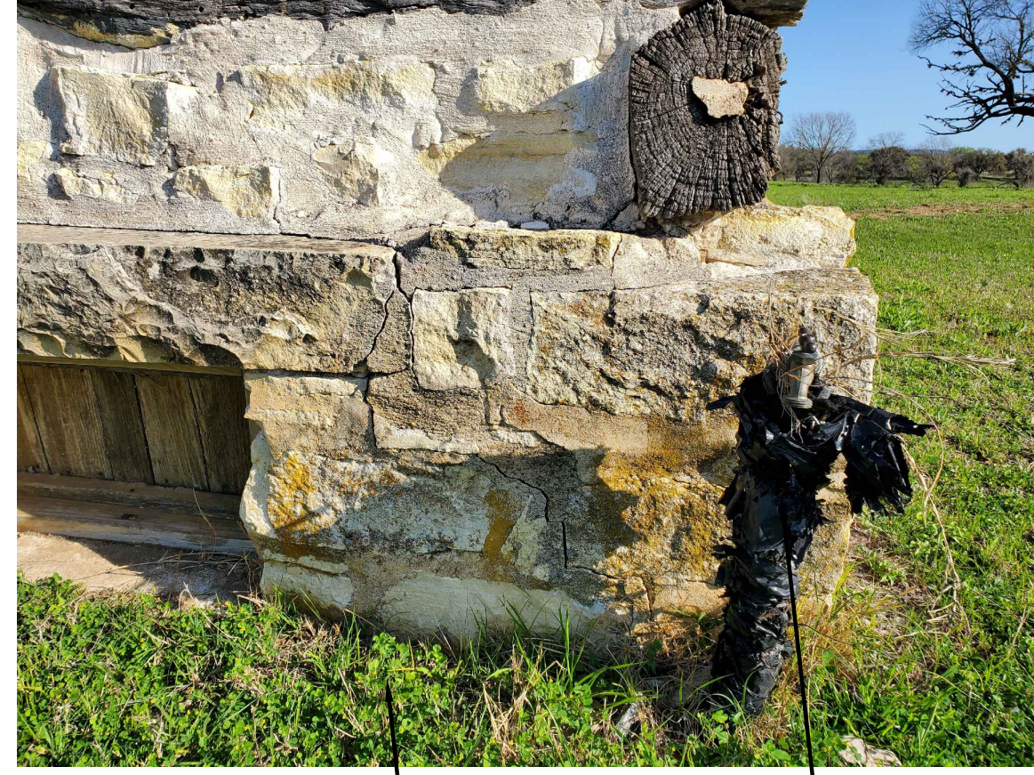
B NORTH CABIN SE CORNER
