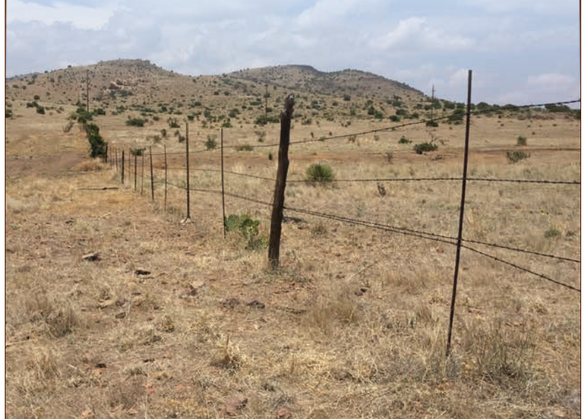
Figure 10. A 4-strand barbed-wire fence is modified by raising the bottom strand from 12 inches above the ground to more than 18 inches.
