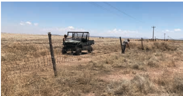
Figure 11. TPWD staff modify a net-wire fence by folding up the bottom to provide at least 18 inches of clearance. Wire is used to tie the bottom half of the fence to fence posts and stays. Tumble weeds are also cleared from the opening.
