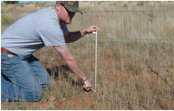
Figure 7. A newly constructed pronghorn-friendly fence is built with three strands of barbed wire and a smooth-wire bottom strand set at about 20 inches above the ground.
