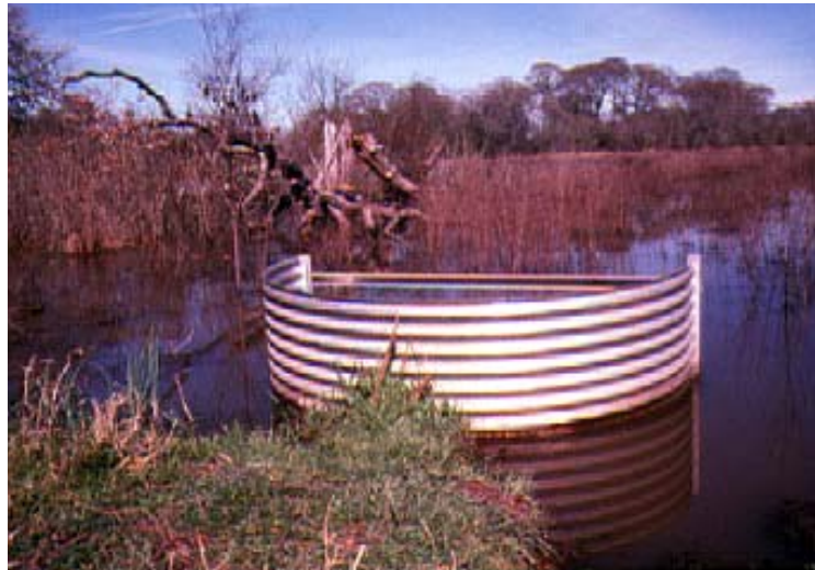
A flashboard riser box attaches to a pipe installed in a levee to create a shallow water wetland for wildlife.
