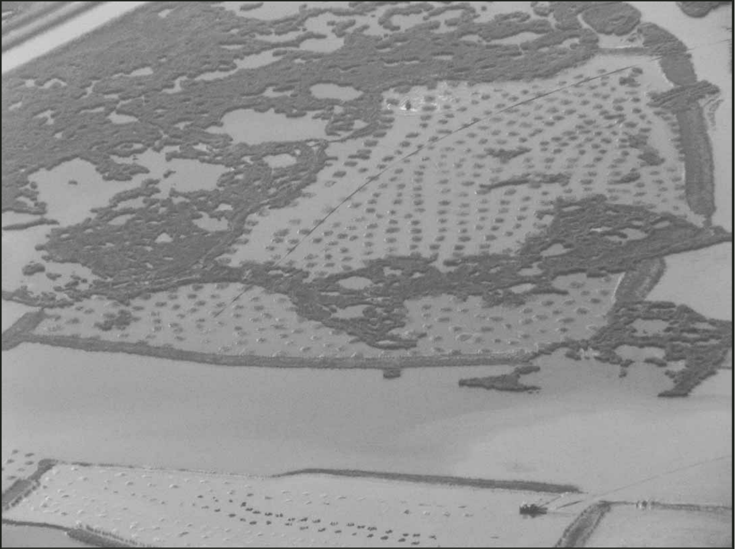
Aerial photo of marsh mounds and terraces during construction.
