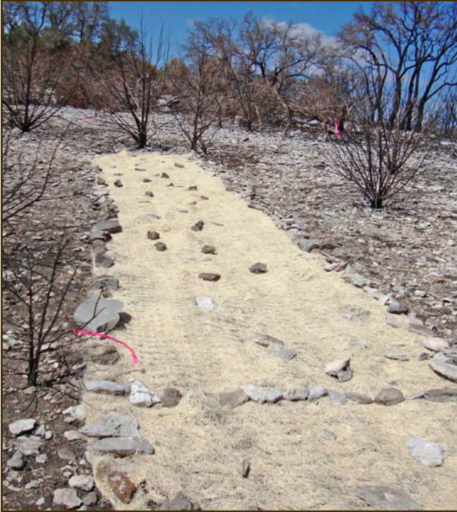
A straw mat was placed on a hillside and seeded in order to slow erosion, trap sediment, and re-establish vegetation.
