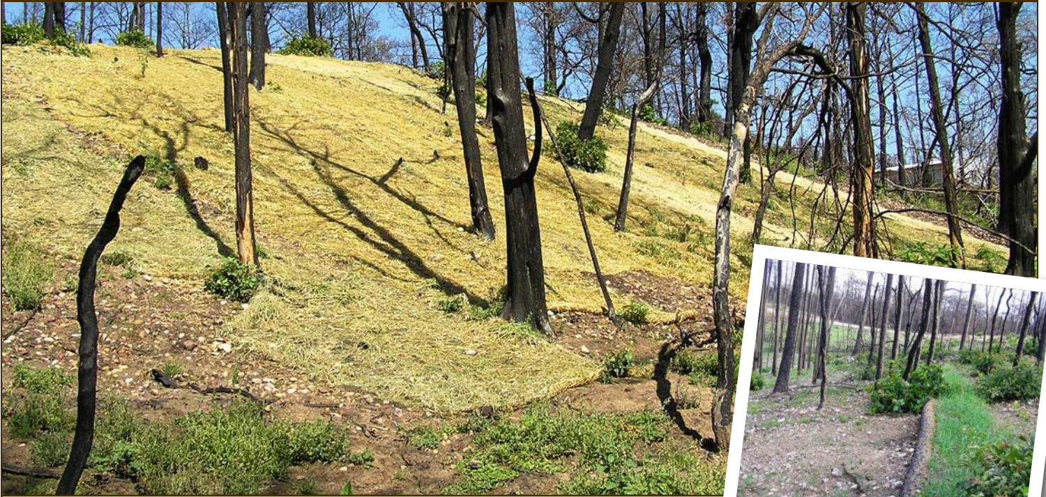
These erosion control mats were used to keep valuable top soil in place following the Bastrop fires.
