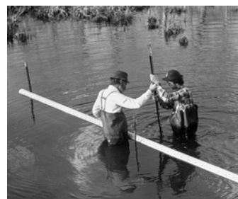
Figure 6. Pipes are situated in the pond with a slight downward pitch toward the outlet end.
