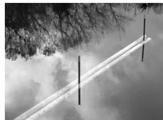
Figure 7. T-posts are suitable supports for the drain pipes.
