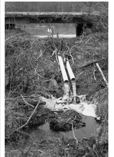
Figure 11. The system is operated by removing the end caps from the drain pipes.
