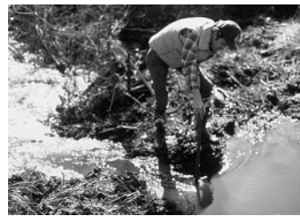
Figure 2. Enlarge the trench and drain water until the desired lower level is reached.
