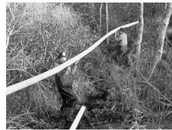
Figure 4. An assembled drain pipe combination is being moved into place.
